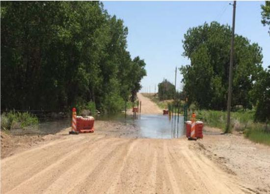
As the water from Crow Creek continues to recede, the county has placed delineator posts every 10' on both sides of the road to channel traffic down to one lane through the crossing as a temporary solution. Signage will warn the traveling public of the possibility of water on the road, and travel on the roadway will be limited to local traffic only.
